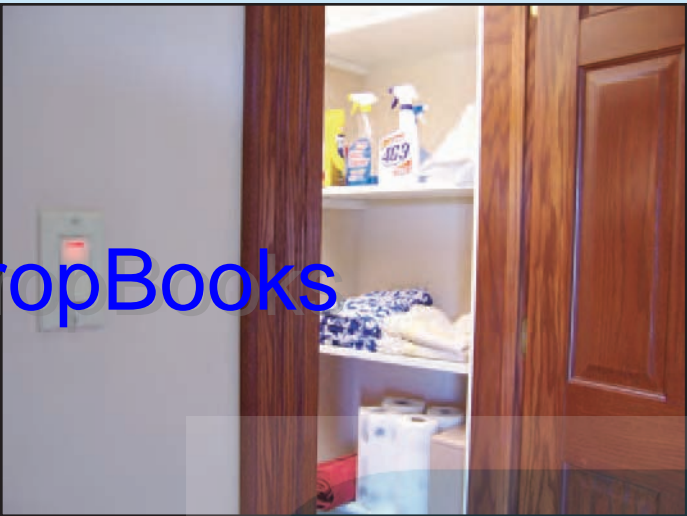
Color Plate 1: This photo shows a closet light switch controlled by a pilot switch. The pilot light in the switch illuminates so that you can tell that the closet light is on, even if the door is closed. The closet is well lit with a 32-watt, four-foot florescent strip fixture. See Chapters 3 and 4 for many good tips on wiring for lighting.
